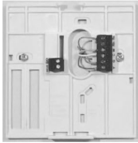
Fig. 2 - Secure Wires to Terminal Strip
